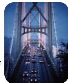
RFID road tolling
